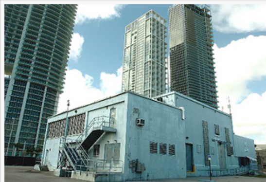
MARICE COHN BAND / MIAMI HERALD STAFF This sewage pump house in Bicentennial Park on Biscayne Boulevard could someday have a complete face lift.
